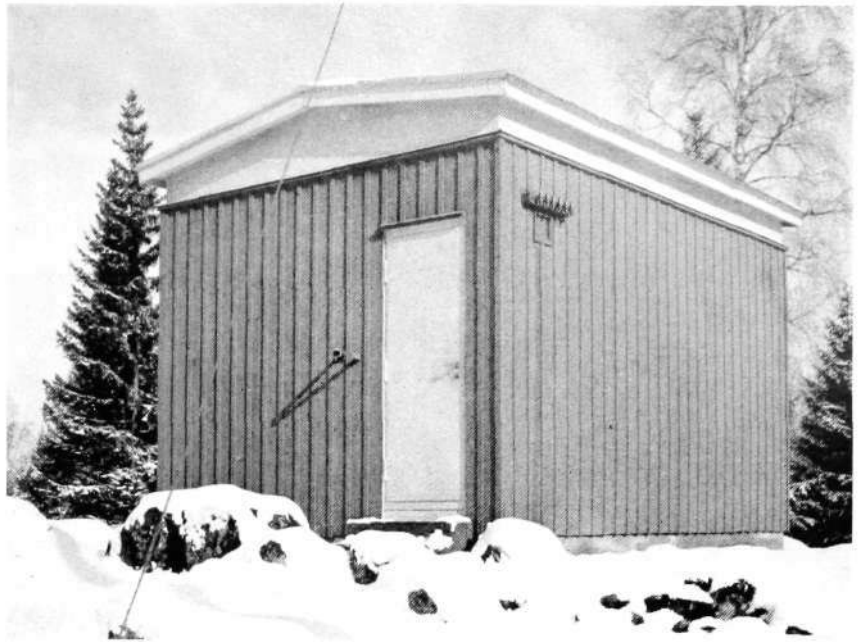
Fig. 16 X 6417 Building for unattended crossbar exchange
