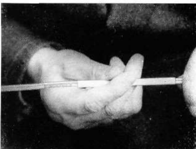
Fig. 3 Splicing PVC wire with a joint sleeve NTA 1401
