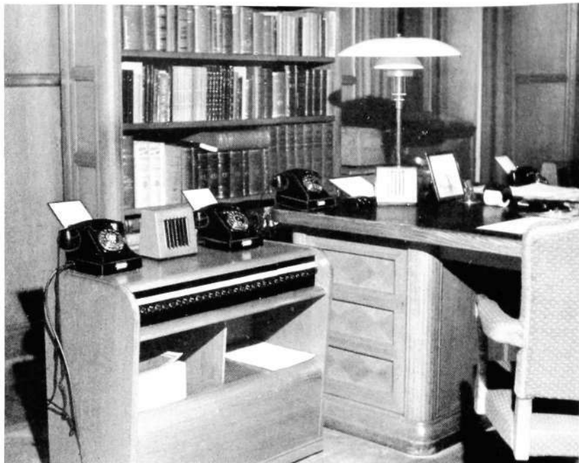
Fig. 5 X 6669 Principal's telephone cabinet, included in the conference telephone system for up to 30 extensions
