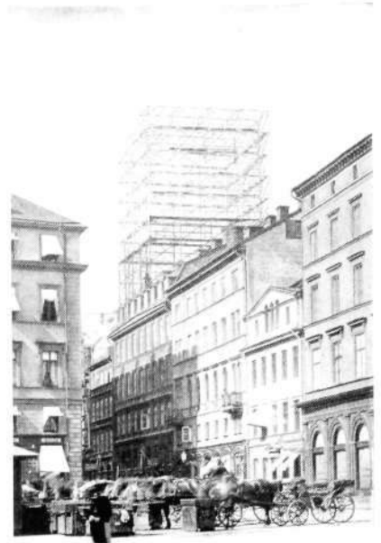
The telephone tower in the original state before the four corner spires were added.
