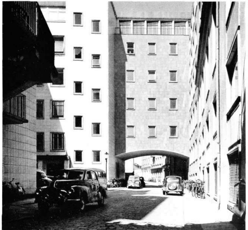
Fig. 1 X 6758 The main exchange premises with the trunk exchange
