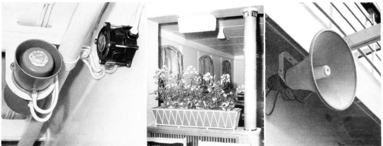
Fig. 3 X 7642 Loudspeakers used left marine loudspeaker RLE 700 , centre pillar loudspeaker, right loudspeaker of reflex type
