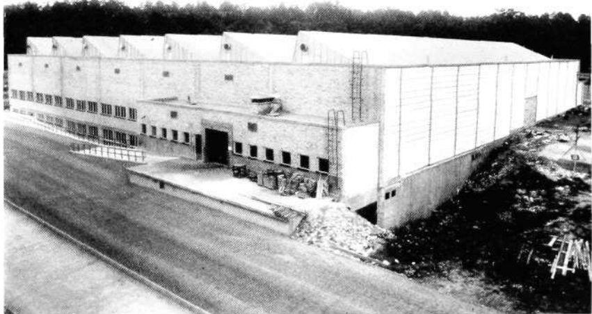
The first extension of the Älvsjö cable shop is 230 ft. in length and 200 ft. in depth. Work is shortly to start on the second stage, which will give the building a frontage of 500 ft.
