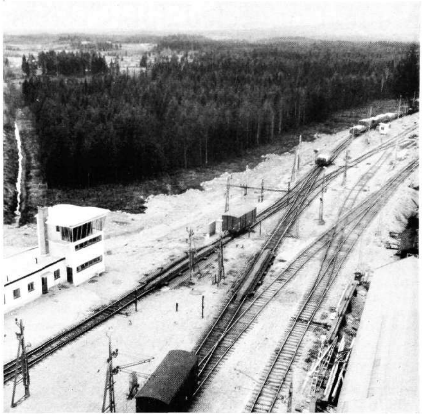
Fig. 8 Automatic shunting from the high hump
