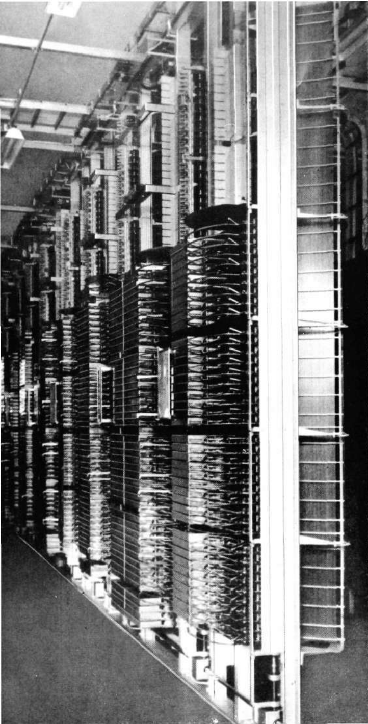
Switchroom in 500-selector exchange at Campo Grande, Brazil
