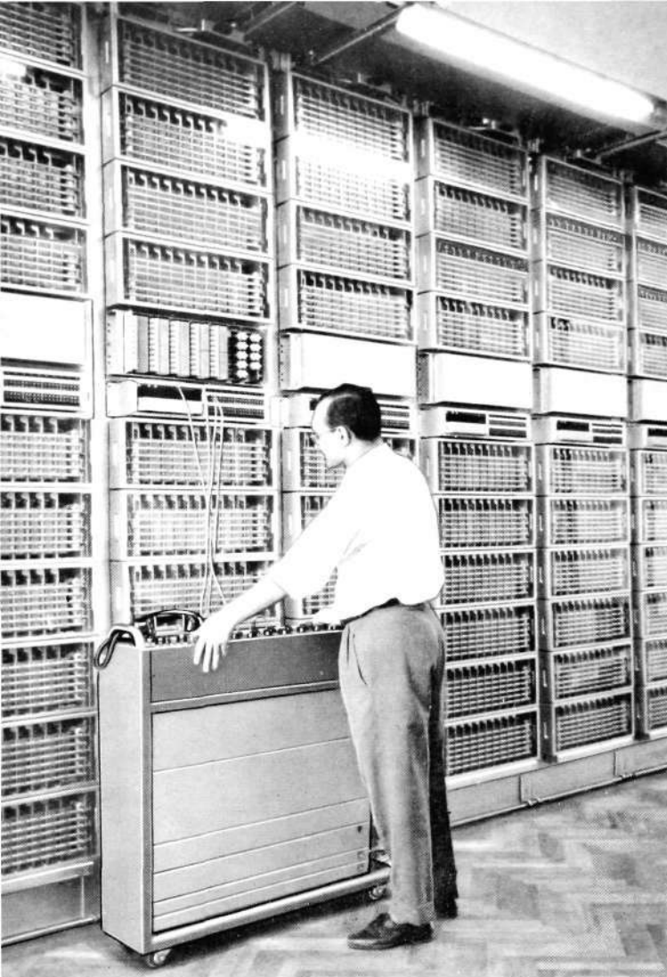
Interior from the new crossbar exchange at Mehalla-El-Kobra, Egypt, United Arab Republic.
