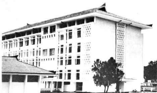
The new crossbar exchange at Padang is housed in a building of rather unusual appearance.
