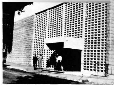
The new exchange building at Reyfoun
