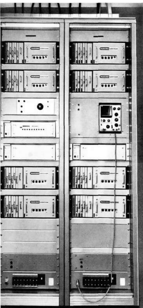
Fig. 9 Distribution equipment for TV installation
