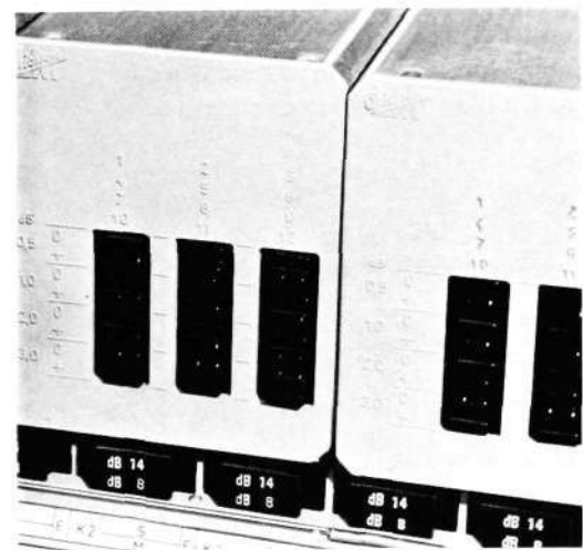
Fig. 11 Channel pads. Arrangement in maintenance strip. The shelf is shown with the cover plates removed
