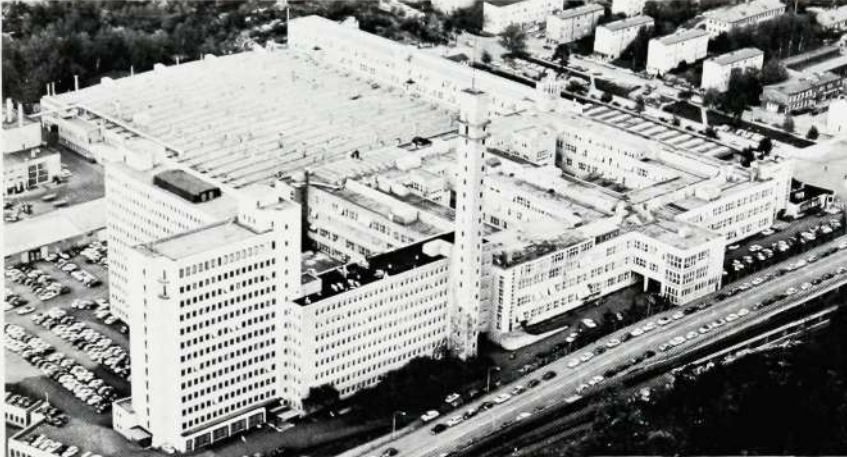
L M Ericsson's head offices and main factory at Midsommarkransen, Stockholm.
