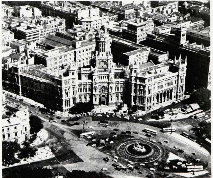
Fig. 1 Palacio de Comunicaciones, Madrid Madrid's telex exchange is installed in this building
