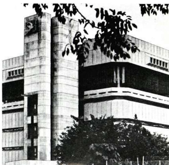
The Orchard Exchange and Engineering Centre, the new telephone exchange at Singapore, for which L M Ericsson supplied its crossbar system ARF 102, was cut over in May.
