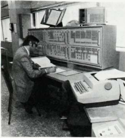
Fig. 8 Control room showing, among other equipment, typewriter terminal for commands
