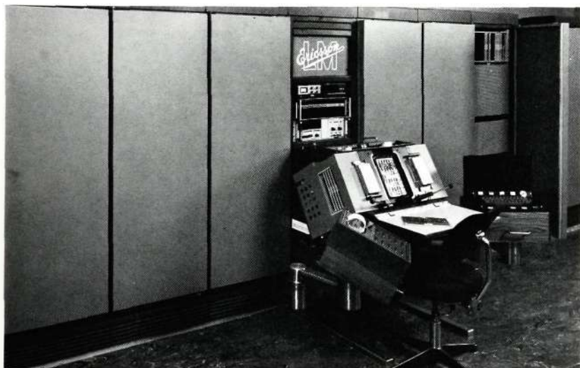
Test position in LM Ericsson's computer-controlled testing system. The positions are controlled by a central computer and each position comprises 5—7 racks containing, among other items, units for logic control, level and time measurement. In front of the racks is seen the test desk with the tester's alphanumerical display terminal and a fixture for objects to be tested — in this case printed circuit boards of type ROE.
