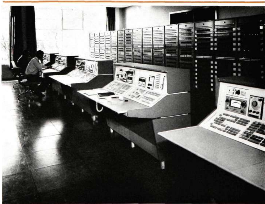
Fig. 8 Test consoles for measurements of the national and international circuits
