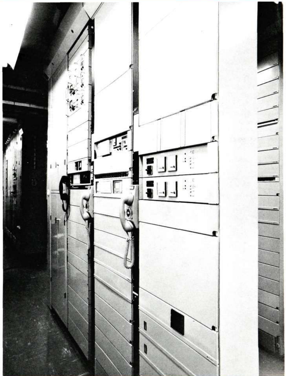
Fig. 8 The terminal station at Nässjö. The newly installed rack is on the right. The racks to the left of this contain earlier generations of 1 M Ericsson 12 MHz and 1.3 MHz systems
