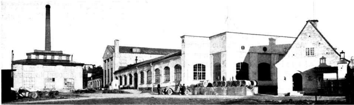
Fig. 6. Another View of the Works.
