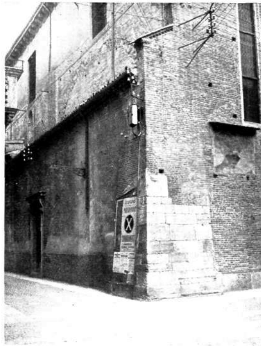
R 310 Fig. 4. 100-pair Distribution Box mounted on Wall of Building.
