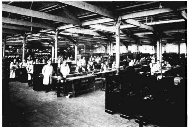
A View of the Switchboard Assembly Shop.
