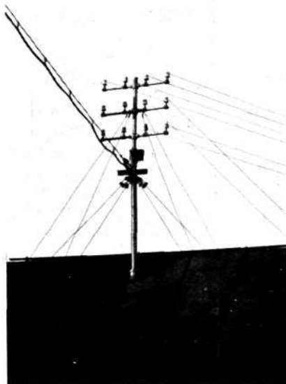
K 11 Fig. 8. Pipe Standard Terminal Box, for Distribution of 10 Open Lines, mounted on Pipe Standard.
