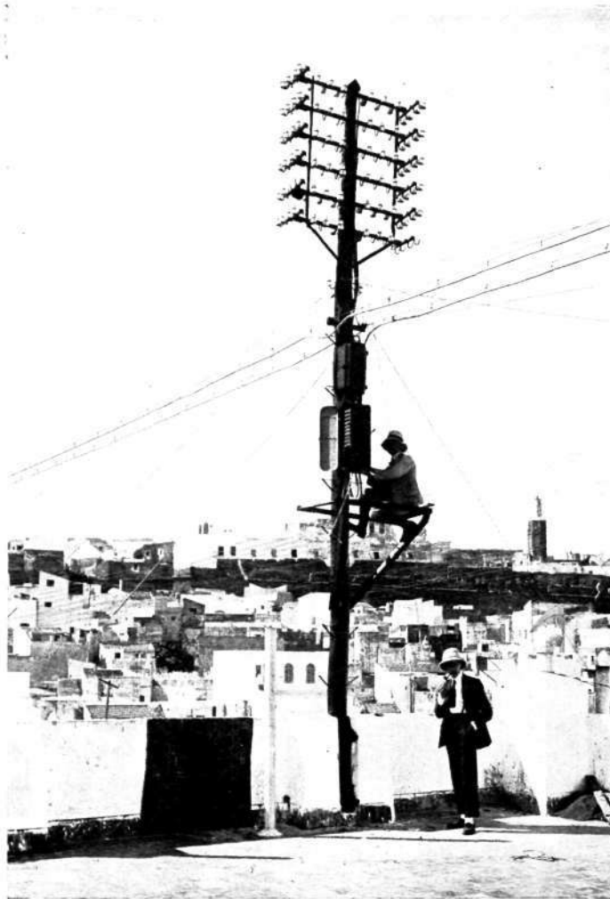
R 234 Fig. 2. 50-pair Distribution Pole erected on a Roof. The larger Cabinet is a Cross Connecting Cabinet for 100 to 130 lines, the smaller one a 50-pair Distribution Cabinet.
