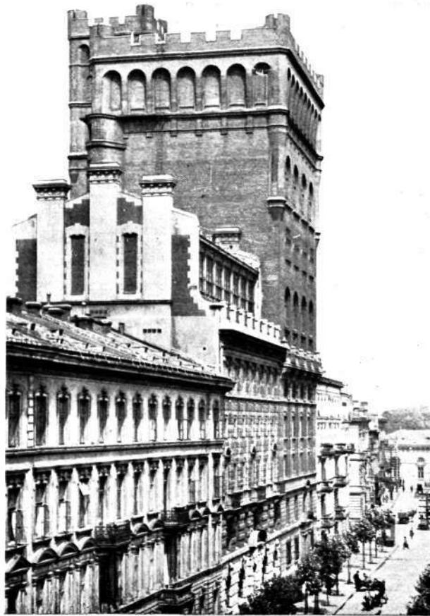
R 258 The Telephone Company's Building in Warsaw.
