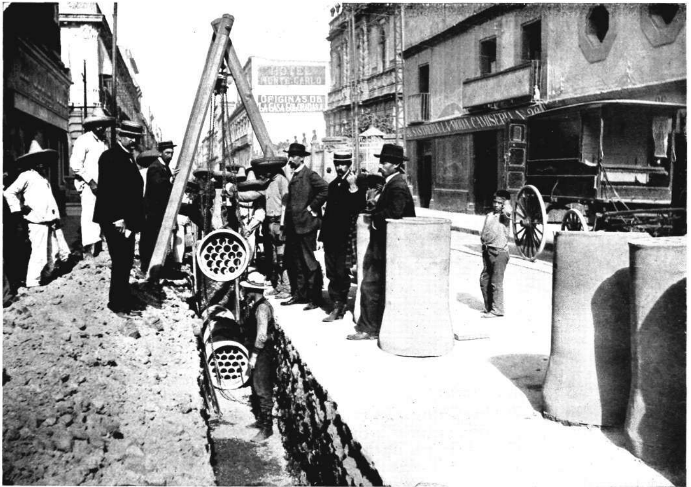
Fig. 1. Laying a Conduit Line in Mexico City.
