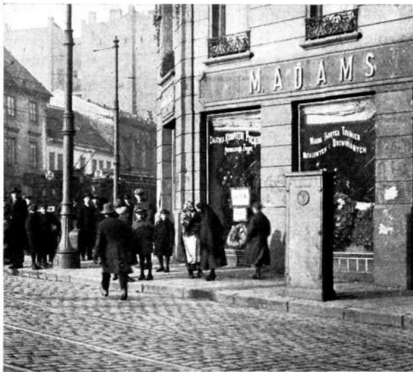
R 277 Fig. 6. Typical Placing of Distribution Cabinet in Warsaw.
