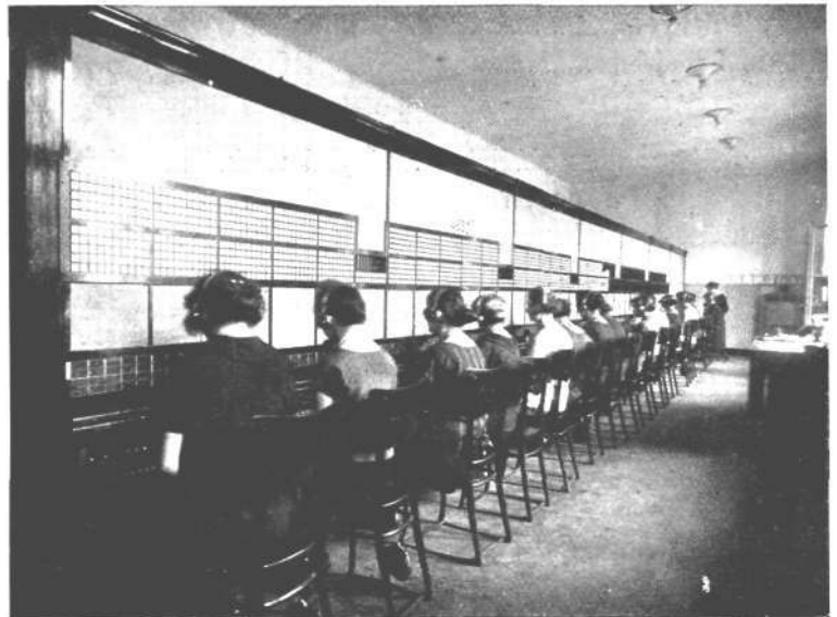
Fig. 3. The Temporary Exchange at Lemberg. Note the Subscribers' Meters over the Local Multiple.
