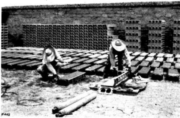
R 442 Fig. 3. Manufacture of Cement Conduits.
