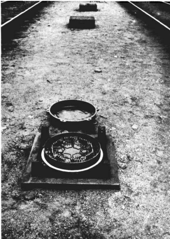
Fig. 8. Cable Distribution Box.
