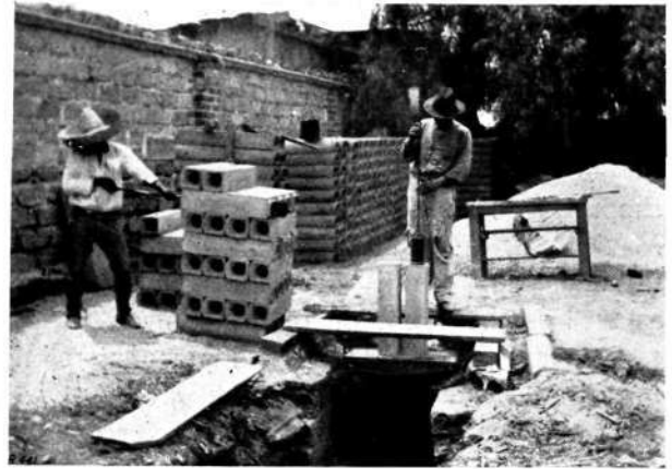
R 441 Fig. 4. Coating Ducts of Cement Conduits with Asphalt.
