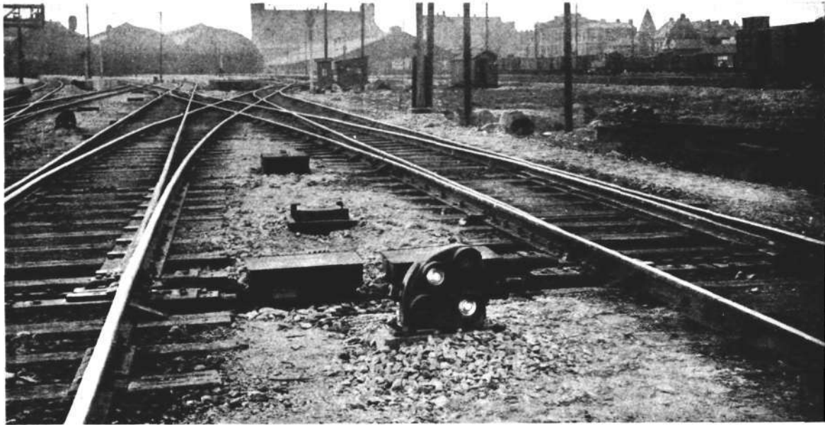
R 404 Fig. 5. Skotch Block Signals. The nearest one indicates »Caution» and the one in the left background »Stop».
