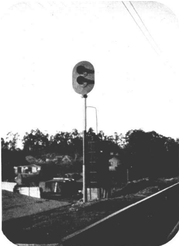
R 681 Fig. 4. Light Signal and Relay Cabinet.
