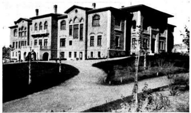
R 600 New Quarters of the National Assembly.
