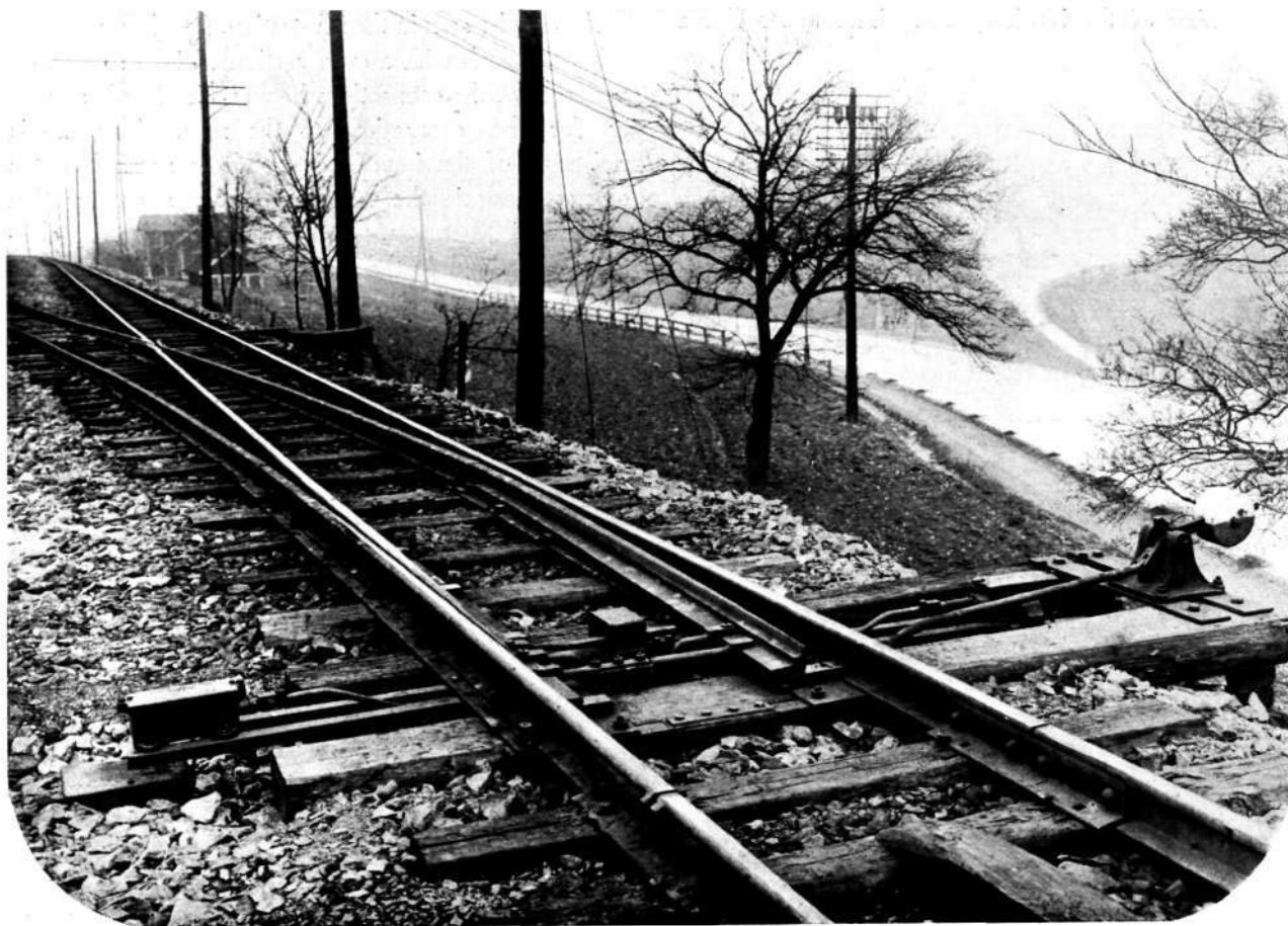
Fig. 9. Point Contacts and Control Lock.
