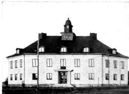
The Clock in the Tower is Actuated by the Same Main Clock as Some Ten Time Recorders.
