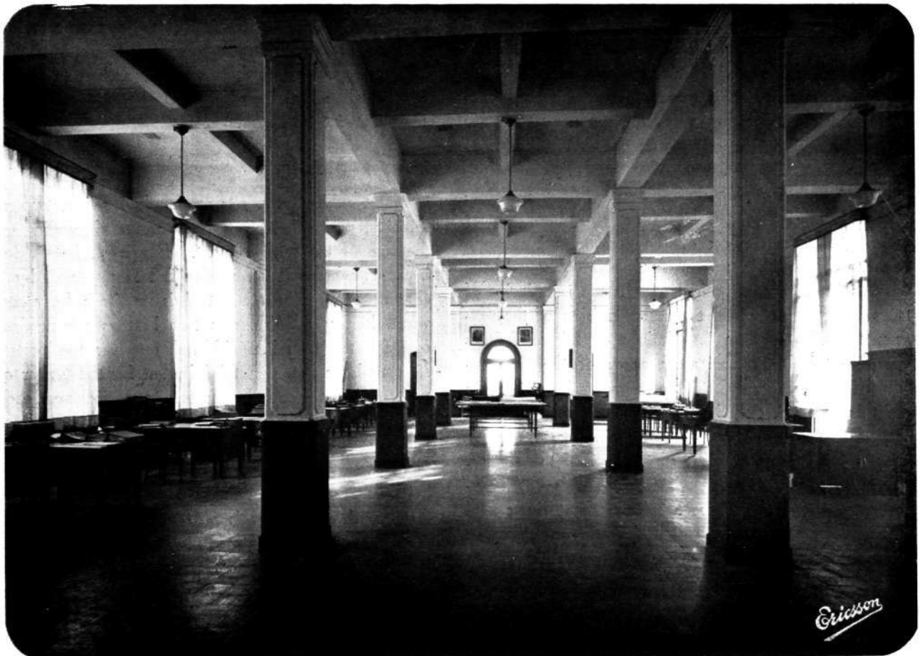
INTERIOR OF ADMINISTRATION BUILDING ON THE PIAZZA NOLANA.
