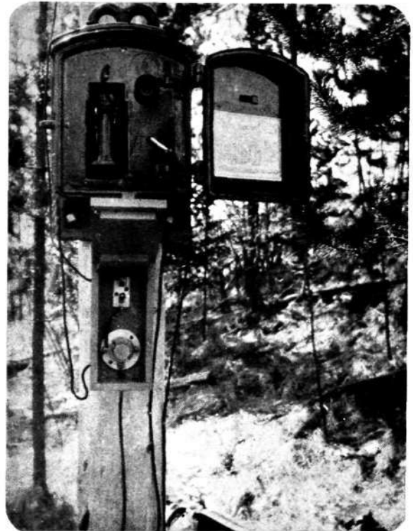
Telephone Cabinet for Fire Alarm Use. (Foto, Can. Forest Service.)
