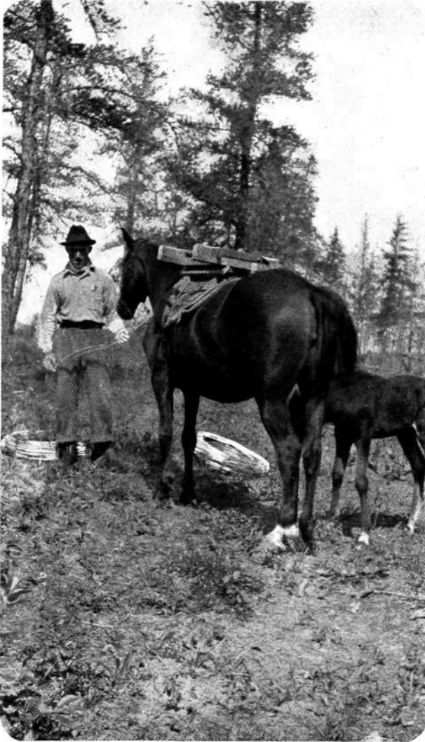
Saddle for Carrying Reels of Telephone Wire used for transportation through forest wilds. (Foto. Can. Forest Service.)
