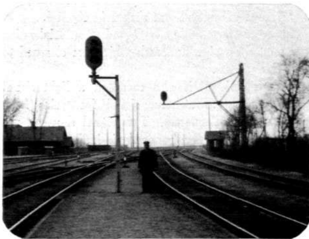
R 1248 Fig. 18. Starting Signals Mounted on Supporting Bracket Arms, Mjølby.
