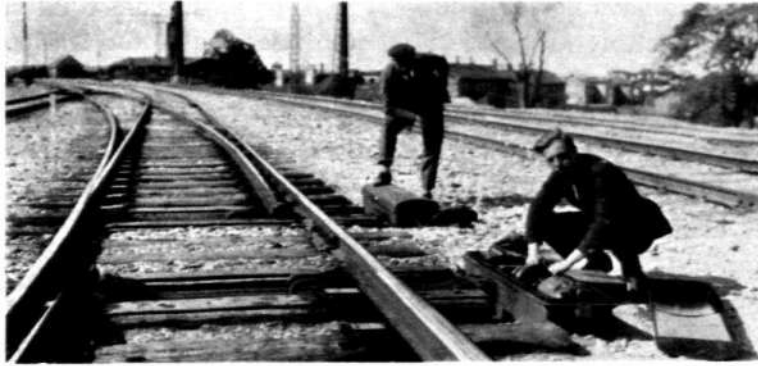
R 1414 Electric Switching Machines with Tongue Control and Enclosed Points Lock.
