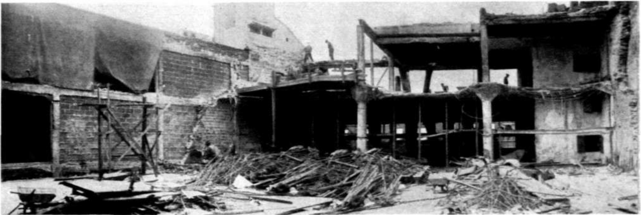
Fig. 2. Even a Concrete Building may be Damaged by Fire if the Fire Department is not Called in Time .
