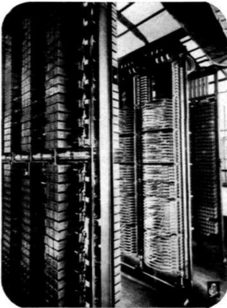
R 1183 Fig. 4. Sequence Switches and Selector Racks.
