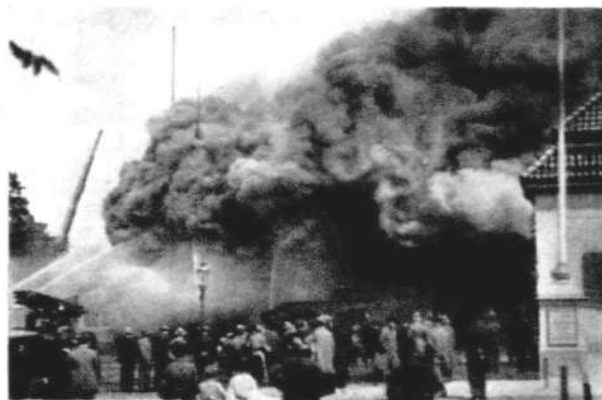
R 1400 Fig. 8. The Djurgård Theatre Fire in Stockholm.
