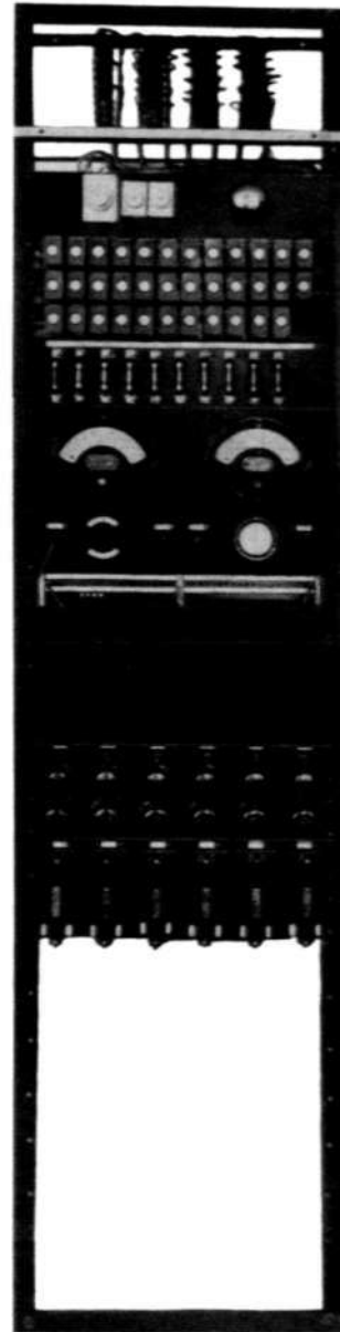
R 1438 Fig. 18. Current Distribution Bay (front view).
