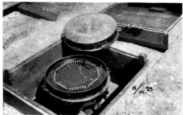
R 1416 Cable Distribution Boxes. Distribution boxes of this type are placed wherever more than three cables are brought together.
