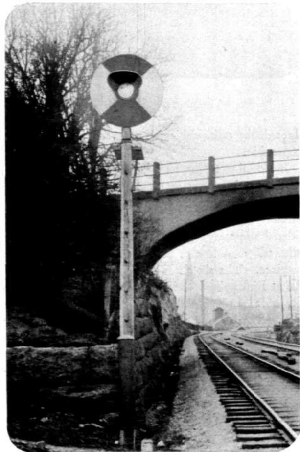
R 1241 Fig. 17. Acetylene Distance Signal at Linköping.
