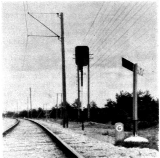
Distance Day Light-Signal. Outgoing Signal eC at Järve.
