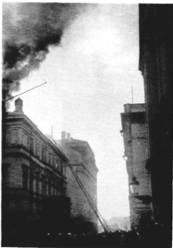
R 1399 Fig. 7. The Fire in Svenska Teatern (the Swedish Theatre) in Stockholm. The theatre building was completely gutted by the fire, the fire department being alarmed too late. Nearly all of the Stockholm theatres are now equipped with Ericsson's automatic fire alarm.
