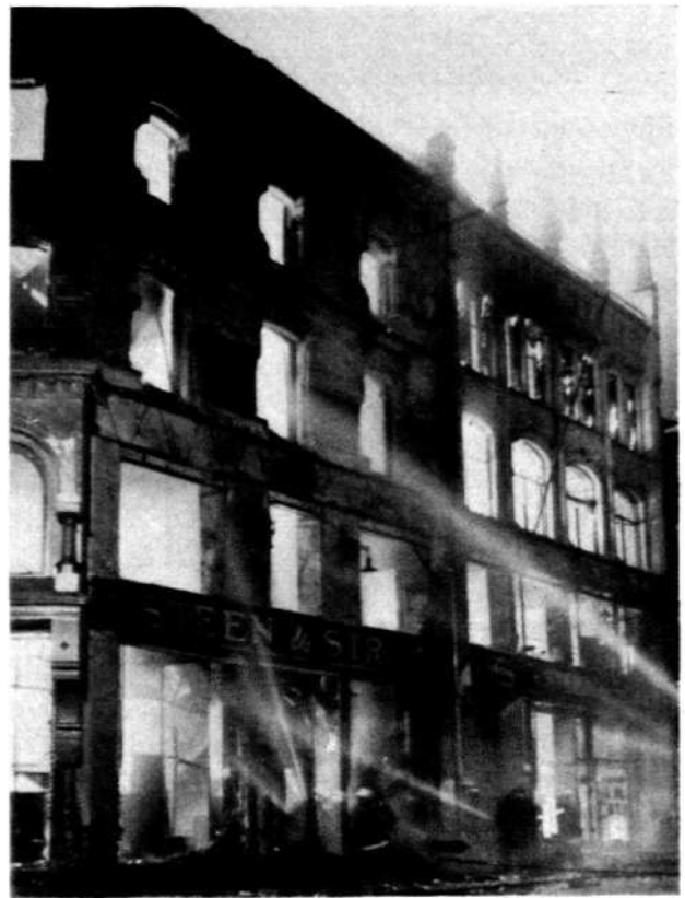
R 1397 Fig. 5. The Million Crown Fire in Steen & Ström's Department Store in Oslo. It would have been a comparatively easy matter to extinguish the fire, which broke out in the basement, had an automatic fire alarm system been installed.
