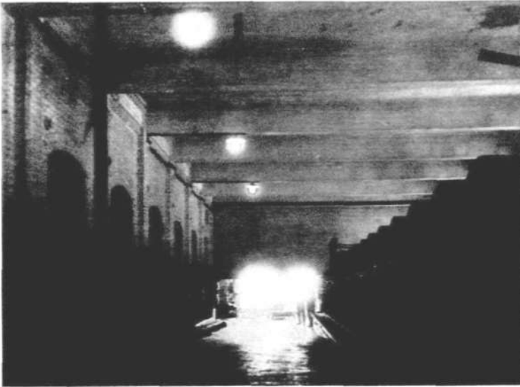
Husum sulphate mill, hall of paper machines.
