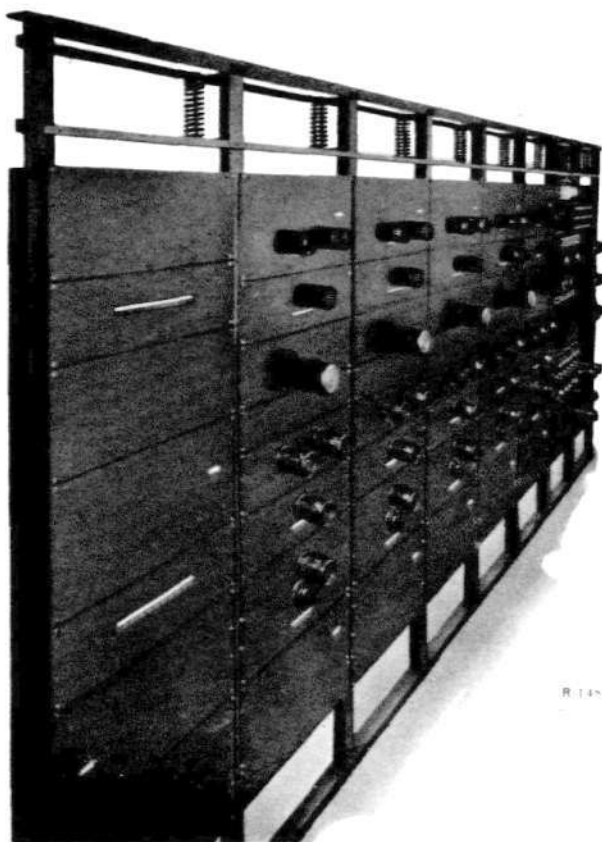
Fig. 24. Carrier Current Telegraph Equipment (front view) at Weltevreden, Java.
