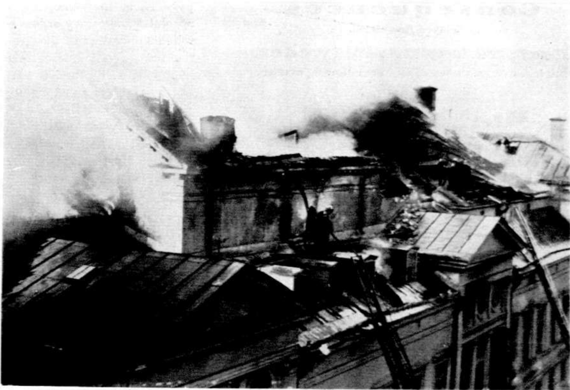
Fig. 20 a. "Svenska Teatern" fire in Stockholm 29.6.1925. Alarm turned in 3.15 a. m. Stage ceiling has collapsed but the ceiling joists over auditorium are still intact.
