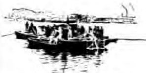
Laying a cable across the river "Göta Älv".
