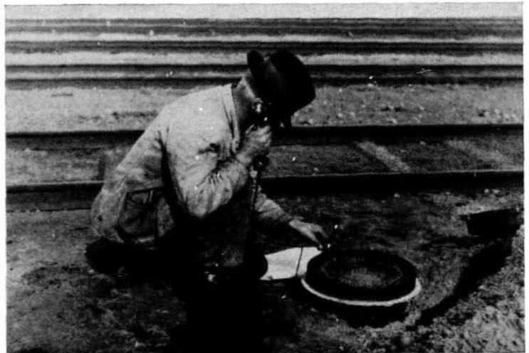
Fig. 25. Testing a cable distribution box.
