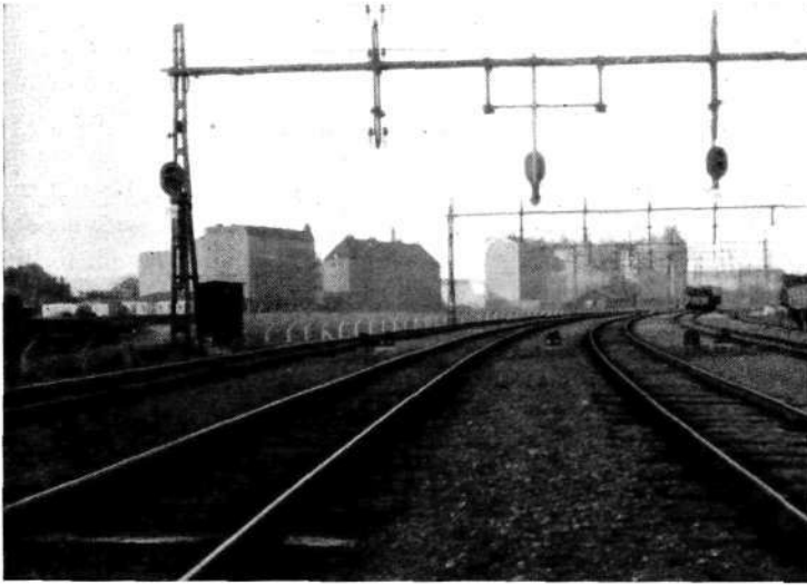
Fig. 10. Incoming and outgoing signals for the Olskroken Lines.
