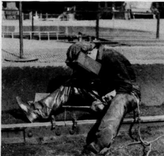
Fig. 23. Welding of rail bond.
