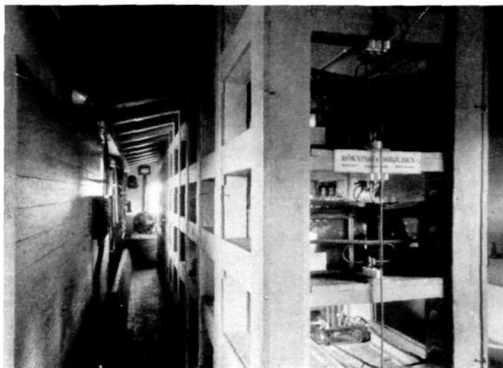
Fig. 16. The first floor of the signal cabin.
