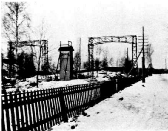
R 4023 Fig. 12. Old fashioned railway-crossing, with a viaduct for the power line.
