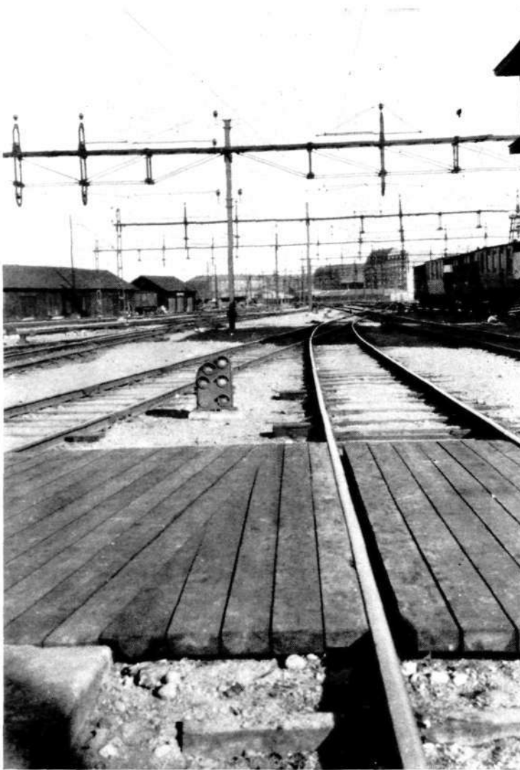
Fig. 12. Dwarf signal at platform track.
