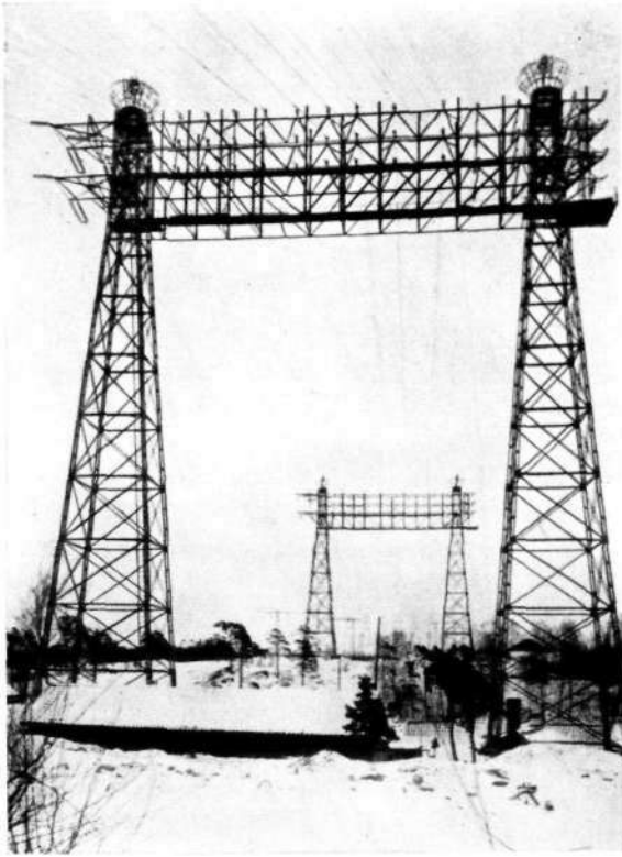
R 4033 Fig. 5. The 130 ft. towers carrying the Trollhättan lines across the Trollhätte Canal.
