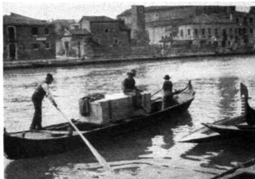
Fig. 5. Transport of material by gondola.
