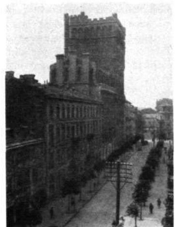
X 3144 The Zielna telephone exchange in Warsaw.
