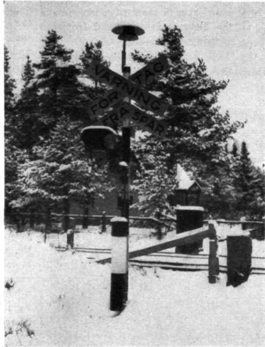
X 1227 Fig. 9. Alarm bell, erected at a railway level-crossing.
