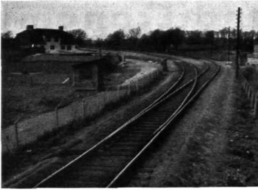
X 1080 Fig. 1. Point on the line operated from a signal cabin at a distance of 1.5 km.
