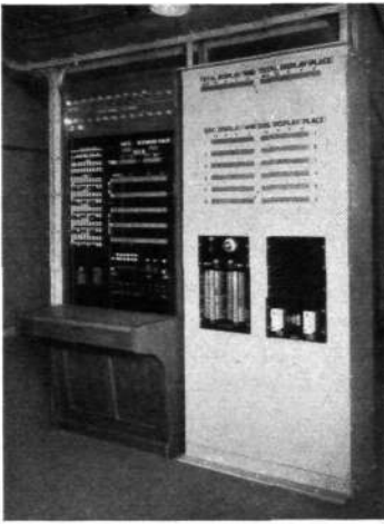
X 3129 Fig. 3. Control switchboard and miniature indicator.
