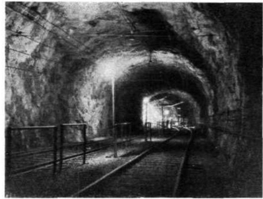
Fig. 2. Part of the concrete tunnel (left), and the rock tunnel.
