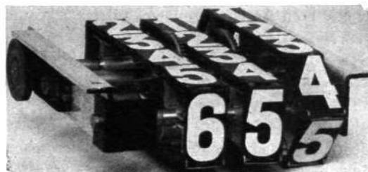
X 1030 Fig. 8. Figure mechanism with three figures, for the difference columns.
