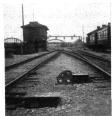
Fig. 2. Dwarf signal and point drive motor.
