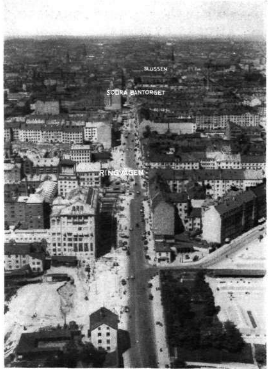
X 1235 Aerial view of southern Stockholm. In the foreground, the opening of the tunnel at Skanstull is seen under construction.
