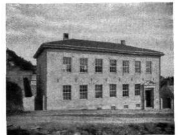
X 3016 The telephone exchange in Hauge-sund.
