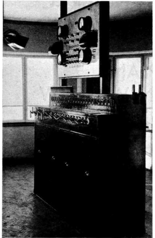
Fig. 2. Interlocking machine with supervisory panel.
