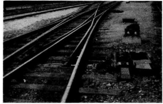
Fig. 21. Double crossing points, with double drive.
