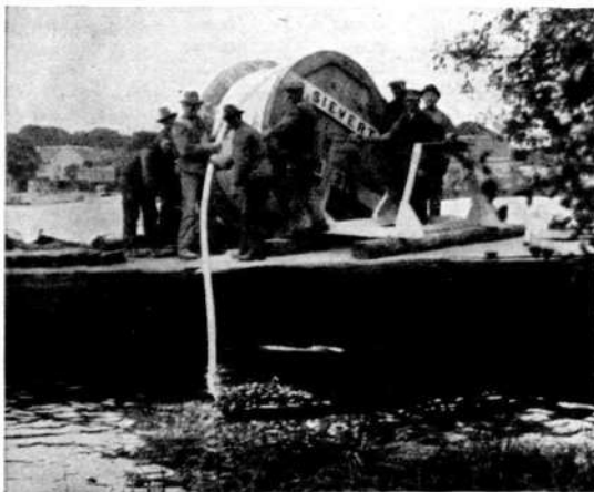
X 1379 Fig. 21. Installation of submarine cable.
