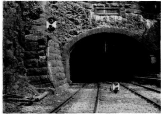
X 1289 Fig. 27. Southern entrance of the tunnel.
