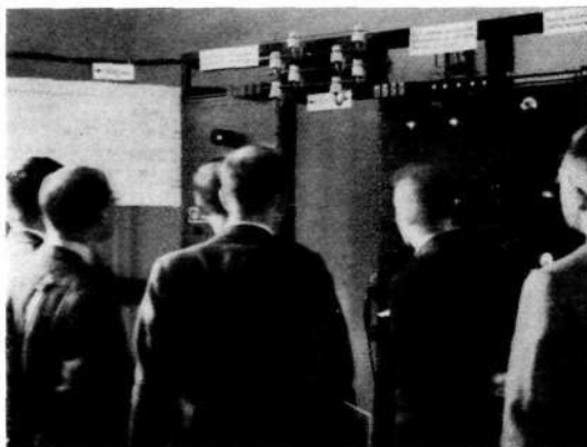
X 1374 Single-channel system shown in operation.
