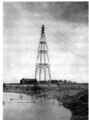
Fig. 3. 70 m crossing pole for 50kV overhead line, near Arnhem.
