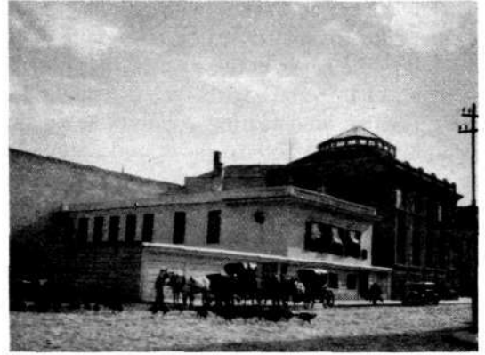
X 1431 The telephone exchange in Izmir, Turkey.
