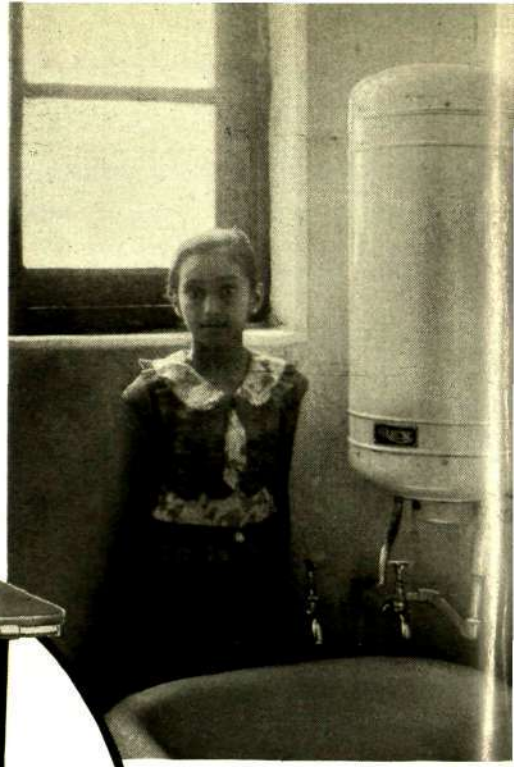
REX hot-water tank in an Indian home in Calcutta
