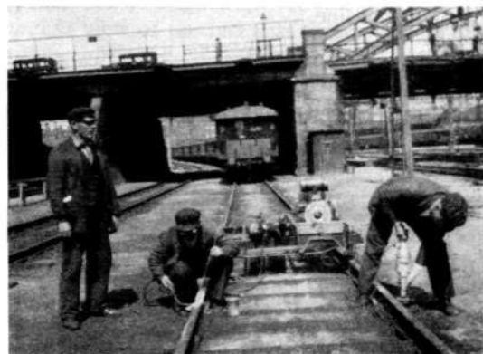
X 1255 Fig. 4. Welding of the connections at the rail joints.
