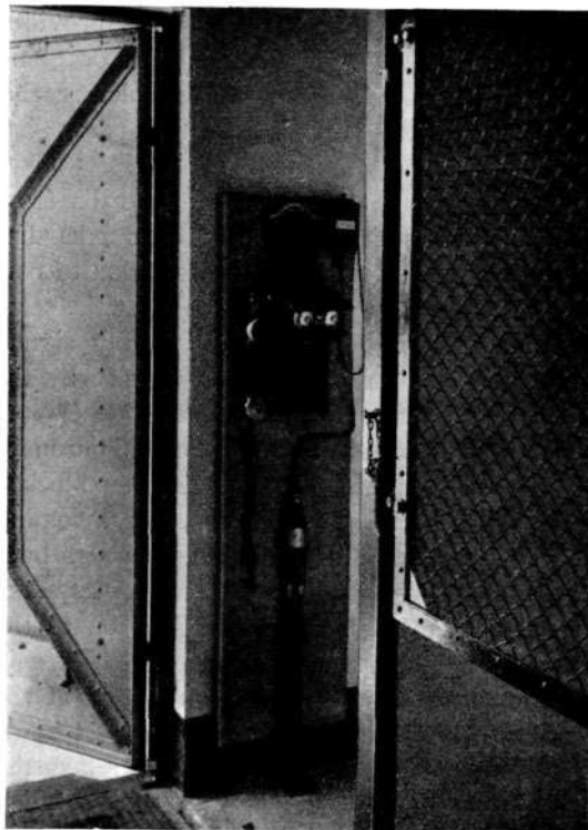
Fig. 12. Telephone instrument, as mounted in a transformer station.
