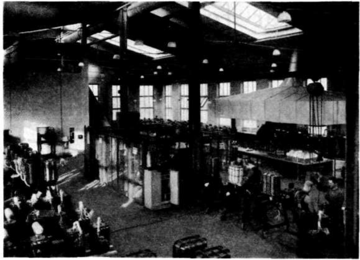
X 3109 Interior of the Ericsson loading-coil works at Älvsjö.
