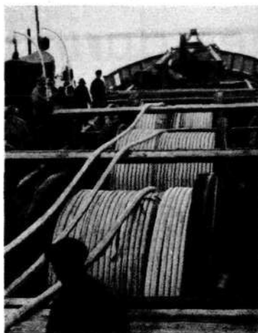
Fig. 3 Laying three 77 kV single-phase cables
