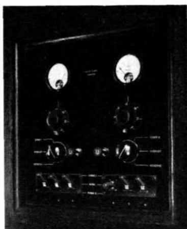
Fig. 7 X 3636 Operating board for remote-control above voltmeter, middle regulating dials and switches for control-impulse sender, below switch for distributing 6 signal groups over two impulse senders
