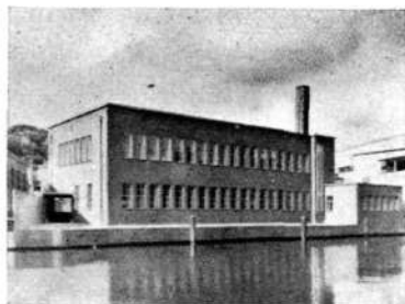
Fig. 1 Schiedam telephone exchange
