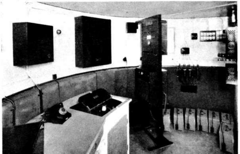
Fig. 5 X 5320 Instrument room left to right: on table talking machine, telephone instrument and gramophone; on wall relay apparatus, private automatic exchange, amplifier rack and charging device; on floor starting apparatuses
