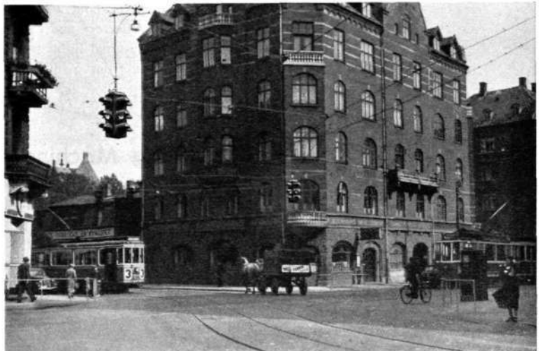
Fig. 1 Street crossing with four-sided traffic signals (to left and in centre) and control box (to right)
