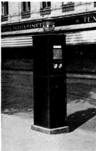
Fig. 3 Control box for traffic regulation in upper part of box are fitted police telephone and fire and police alarm
