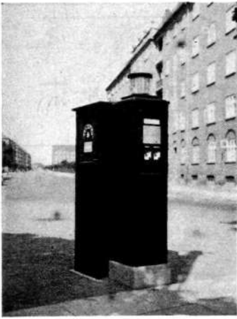
Fig. 4 X 3253 Combined alarm box and telephone cabin incorporating traffic-regulating machine
